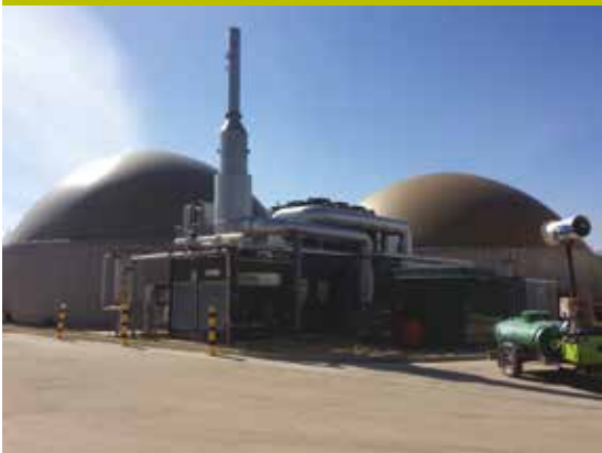
Figure 16: Commercial anaerobic digestion plant converting organic waste into methane for energy and digestate
